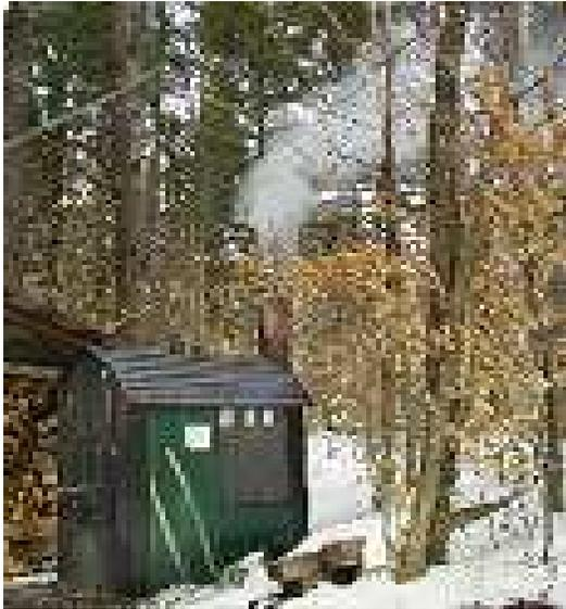
**Two-stage, downdraft gasification heater (low-mass boiler) with thermal storage**
